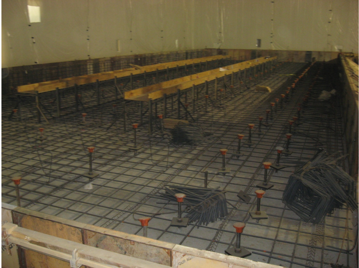
Figure 8 - Hollow Bar Micropiles Prior to Pouring Equipment Pads
